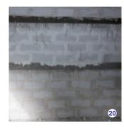
On the **corner and side wall bindings**, masonry should be cross-sectional, so the walls can have better mutual support (see Images 11, 12). The **vertical joints** are not bonded to each other when they have groove (male-female), but there is a need for bonding where **THRAKON** blocks are cut (see image 9).
