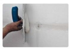
After the installation of plastic anchors proceed in the putty to ensure the surface remains flat.
