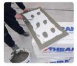
The method of application of adhesion material and the thickness of coat are depending on defects of substrate.
